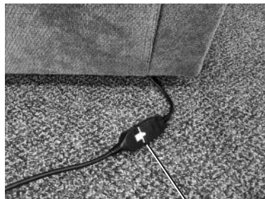
Power Transformer Connection
